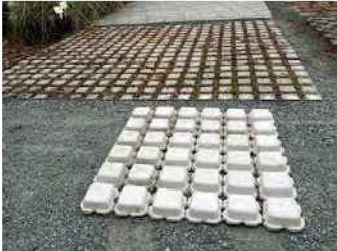
CONCRETE GRASS PAVERS SET ON MIN. 6-INCHES COMPACTED AGGREGATE BASE COURSE
