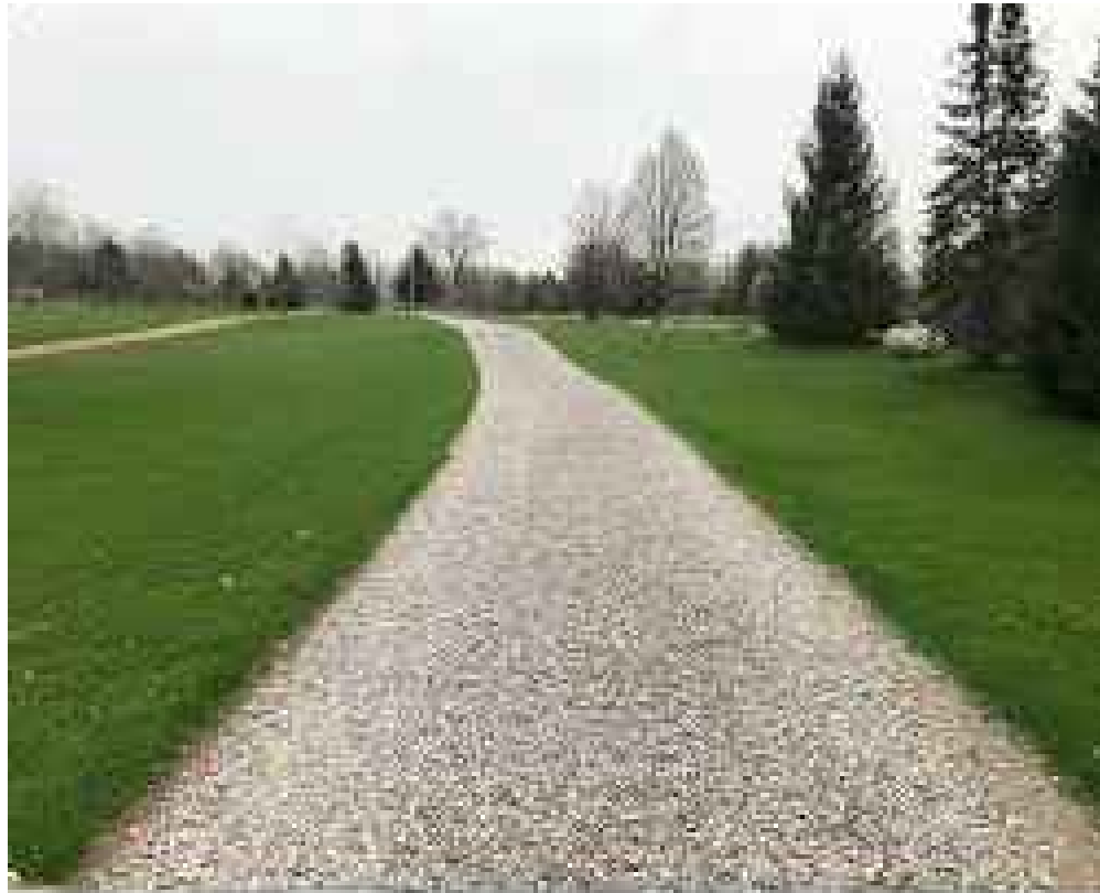
10-INCH THICK COMPACTED AGGREGATE BASE COURSE WITH WOVEN GEOTEXTILE FABRIC INSTALLED BETWEEN SUBGRADE AND AGGREGATE BASE COURSE (ABC)
