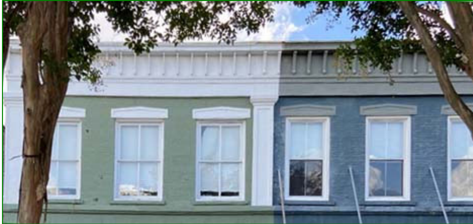
Figure 28. Examples of Upper story windows; windows in the left half of the building are original; the windows in the right half of the building are appropriate replacements.
