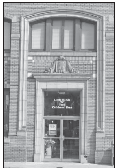
The historic windows of this building on Congress Street have been appropriately retained along with the lintels; all of which are character-defining features of this building.
