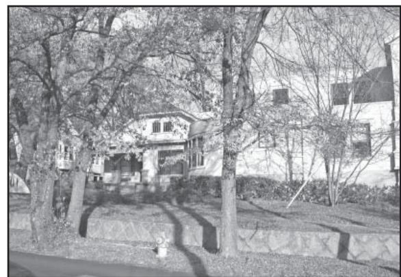
This clipped roof Bungalow in Stone Mountain, Georgia, was inappropriately rehabilitated for office use circa 2000. Inappropriate alterations include: 1) stucco was applied over the historic cladding; 2) the front porch was infilled; and 3) an addition double the size of the original house was added to the side and stepped forward in front of the original front facade.
