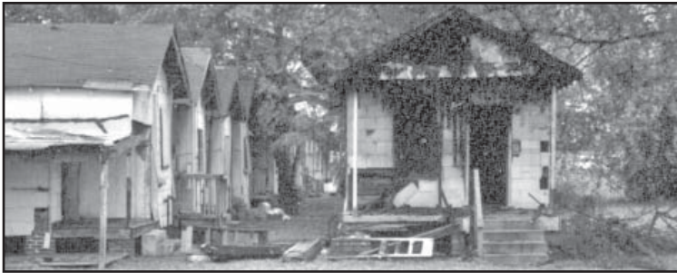
This shotgun house type in Columbus, Georgia, was abandoned and is in the process of demolition-by-neglect. Demolition-by-neglect attracts vandals which often may lead to arson, as in this case. This can easily destroy a whole historic area.
