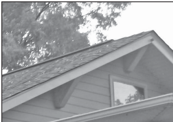
This bungalow in Calhoun, Georgia has had its knee braces inappropriately replaced with triangular pieces of solid wood. This has altered the integrity of the Craftsman style associated with this bungalow and has detracted from the ability of the resource to convey appropriate feeling and association for its period of significance.
