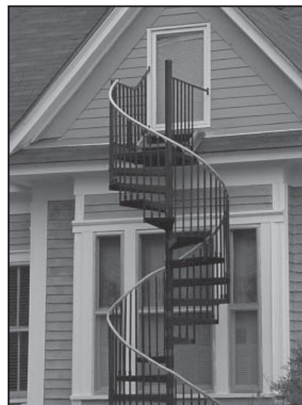
This fire escape was inappropriately added to a prominent flush gable in northern Georgia. Fire escapes, whenever feasible, should be placed so as not to obstruct significant features of a historic resource.
