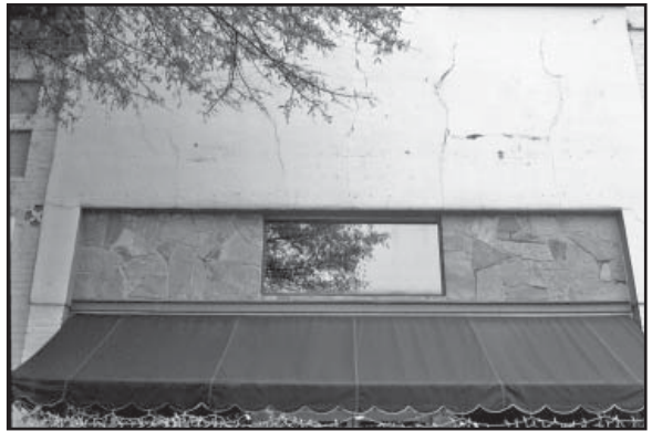
This transom has been inappropriately infilled with faux stonework.
