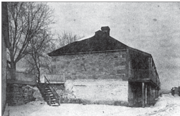
(a) and (b). Two views of the Officers' Quarters at Fort Snelling (ca. 1885 to 1900) not only provide information on the materials and form of the historic block, they document the wooden walkways and other landscape features such as stairs, railings, and tree placement. Historical and pictorial evidence would need to be combined with specific physical evidence in order to make the case for Reconstruction as a treatment.
