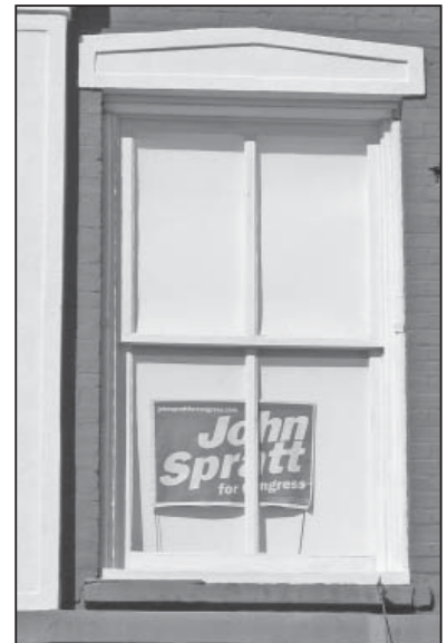
The historic windows of this building on Congress Street have been appropriately retained along with the lintels; all of which are character-defining features of this building.
