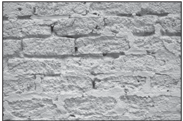
This is an example of what happens when masonry is cleaned improperly by sandblasting of the surface. Masonry has a protective "skin" which protects against infiltration of moisture. If this skin is removed, as is the case with sandblasting, the brick can no longer repel moisture.
