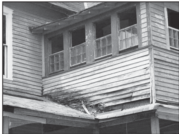
If the flashing and cladding had been periodically maintained the deterioration of the wraparound porch roof and the exterior cladding would have been halted. Extensive in-kind replacement is needed for this south Georgia residence which will be less cost effective than regular maintenance would have been.
