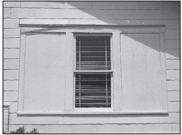
This window was originally a tripartite window a unique design element on this residence that has been obscured by exterior grade plywood creating a loss of integrity for this historic resource in south Georgia. The infill of extant historic window or door openings is not appropriate.
